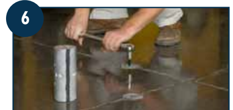
6 SD Joint Stabilizers are expanded by torquing to 85 ft. lbs.
