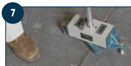
7 Deflection is again measured and recorded to confirm success.(optional)
