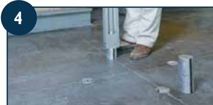
4 SD Joint Stabilizers are installed.
