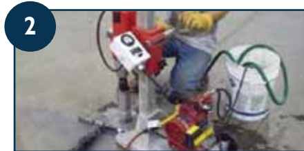
2 Certified installers use specialized equipment to drill core holes.
