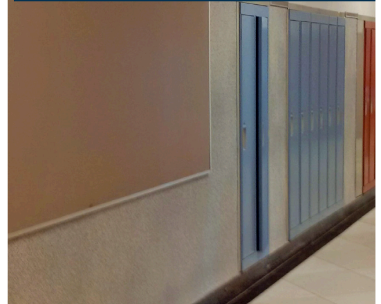
AREA: HALLWAY WALLS
